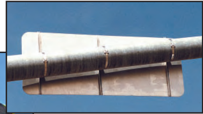
Mast Arm Sign Installation
